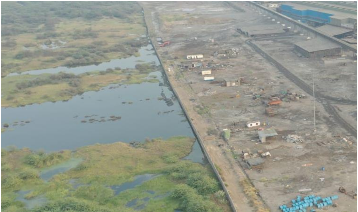
Photograph of Water Accumulation in Reserve Forest Area (Annexure-C1)
