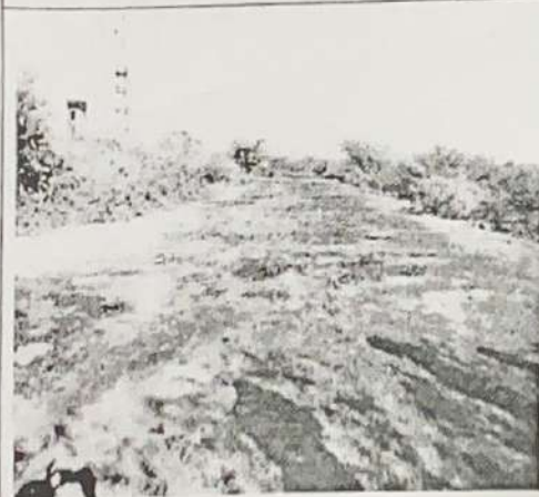
copper slag was utilized in constructed road near GMB Port area
