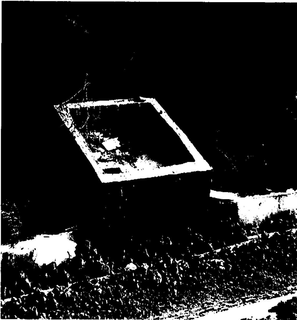
Lechate collection sump of SLF VII
